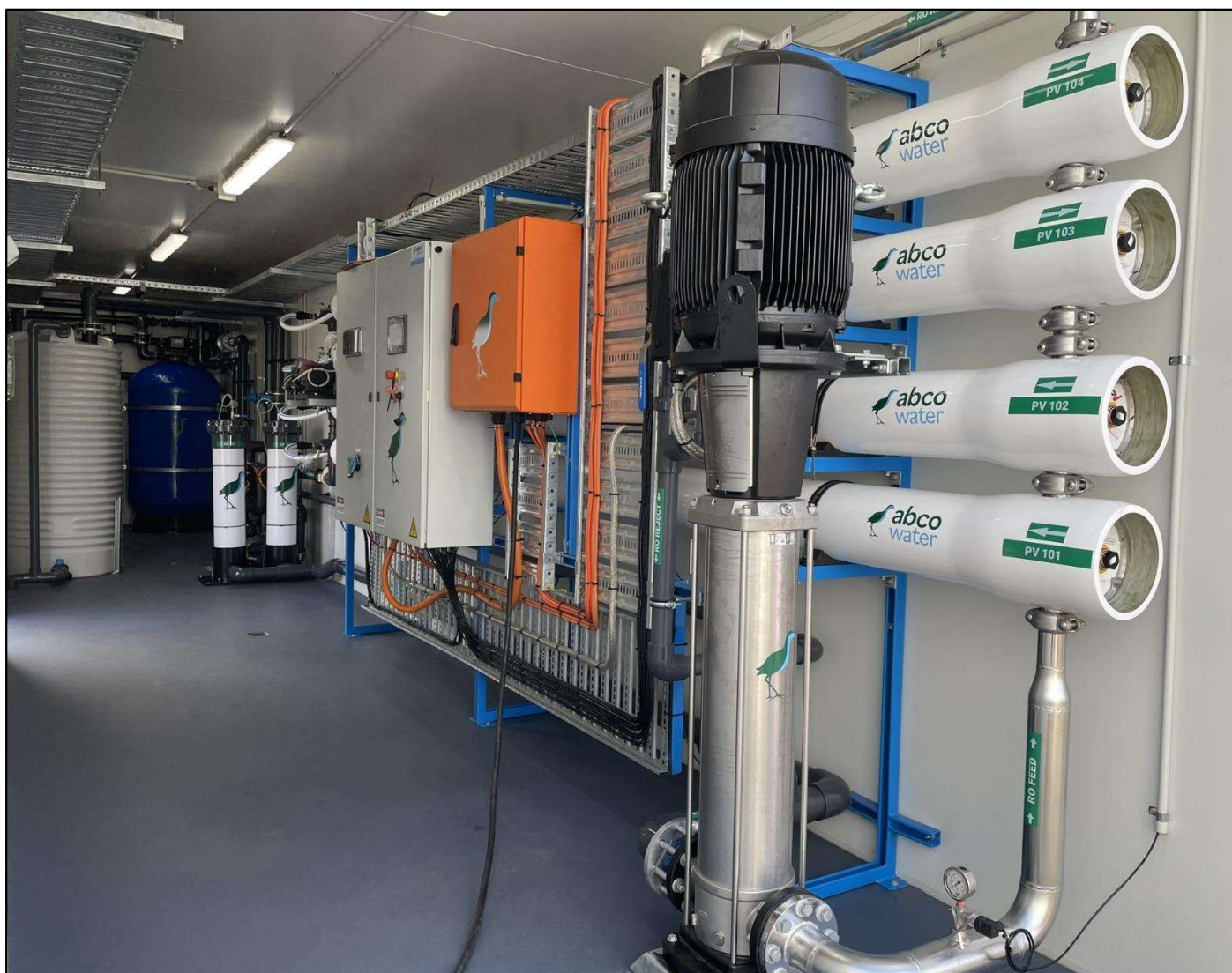
ABCO 480 m 3 /day containerised RO plant
