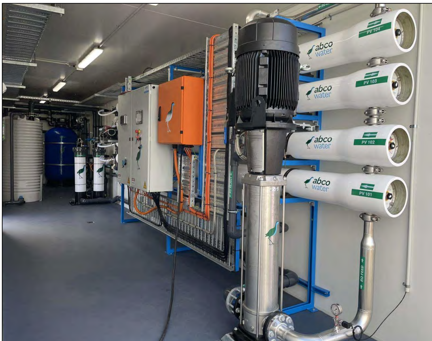
ABCO 480 m 3 /day containerised RO plant
