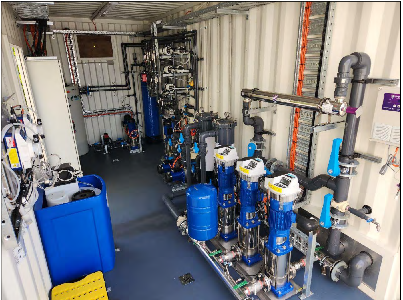
ABCO 24 m 3 /day containerised RO plant
